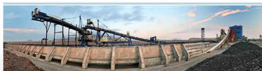
MATERIAL HANDLING, STACKING & RECLAIMING OF SANGAN IRON ORE CONCENTRATE PLANT (EPC)
